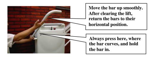
• The platform can be released manually by raising it to its vertical position to allow free passage on the stairs.
