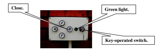
K. Before leaving the lift, put the key into the key-operated switch on the nearest operating panel and turn it until the green lamp goes out. <u>The lift is now locked.</u>
